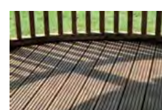
Raised Timber Floor
